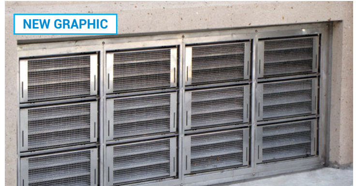
Engineered flood vents are part of a wet floodproofing strategy.
