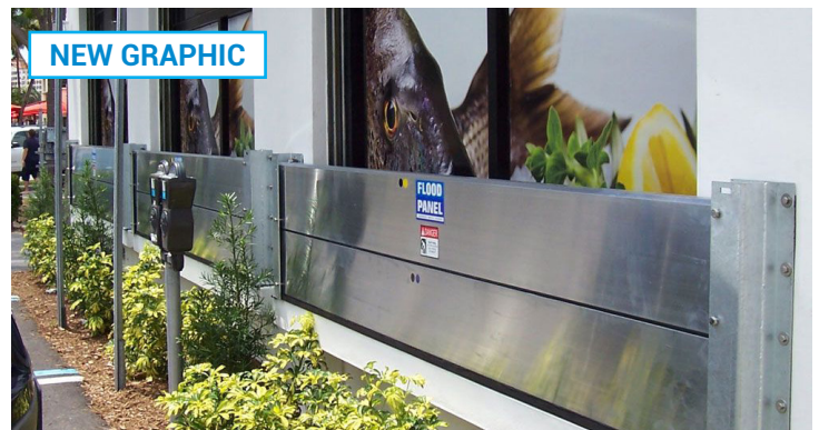
Deployable flood barriers are part of a dry floodproofing strategy.
